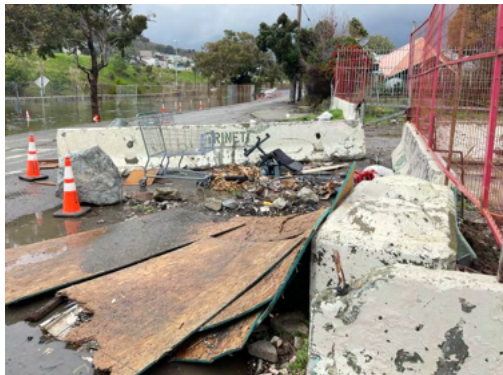
Trash and debris sit in floodwaters at the entrance to the Bayview Vehicle Triage Center in San Francisco. The situation forced the city to bulldoze a new entrance to the facility. (Joe Dworetzky/Bay City News Foundation)
